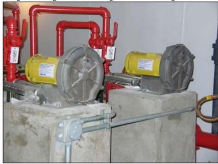
Each lagoon has a separate pipe to the blower building with an isolation valve and a Pressure and Vacuum Relief Valve with Flame Arrester used to protect the lagoon from an overpressure condition. Typically, lagoons have a maximum operating pressure of 2" WC or 50 mm/WC. We provide redundant blowers that can be selected to run separately, together, or on a lead/lag basis.
