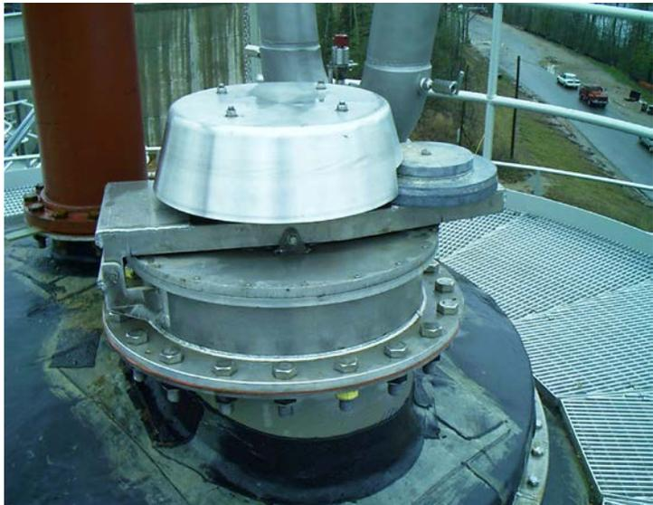
Take for instance the Newtown Creek Wastewater Treatment Plant in New York. During the initial testing phase, an overflow of sludge and foam caused clogging of the flame arresters and PVR valves. The digesters were subsequently damaged because the pressures increased above a safe level. New York City Department of Environmental Protection (NY DEP) contacted Varec Biogas for assistance.
